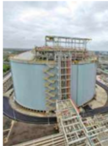
Dahej LNG terminal ranks as the sixth largest globally.
